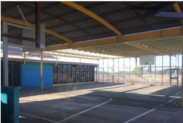
Basketball court and outdoor areas are completed.
