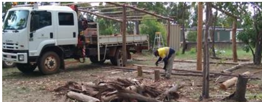
Building a structure at the Gulkala site for the Garma Festival
