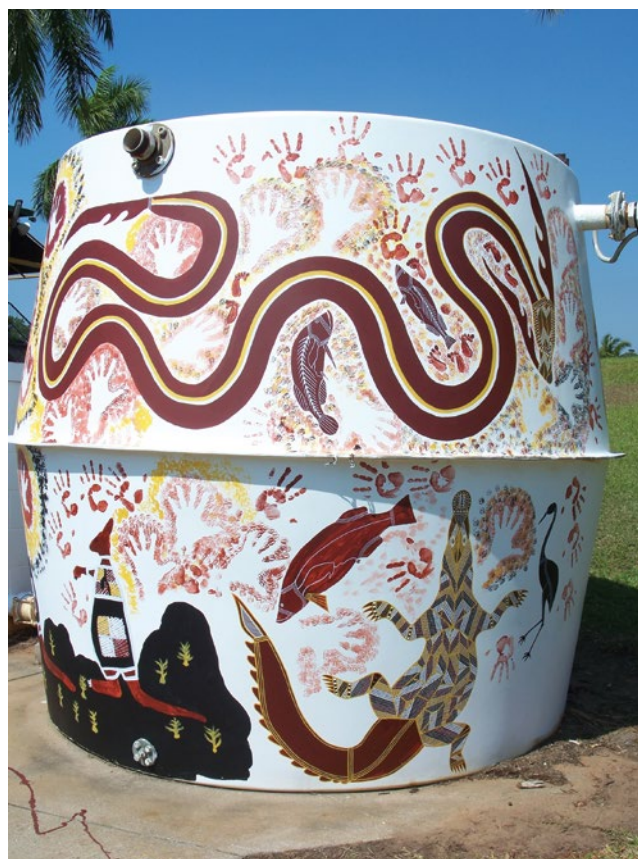
Hockey NT Project – water tank
