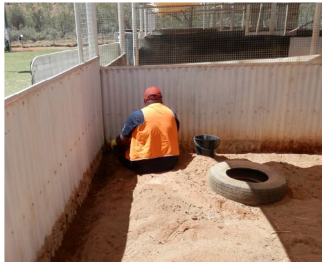
Repairs, maintenance and painting stables
