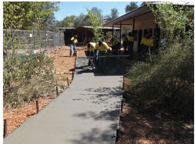
Building at CAAAPU with prisoners
