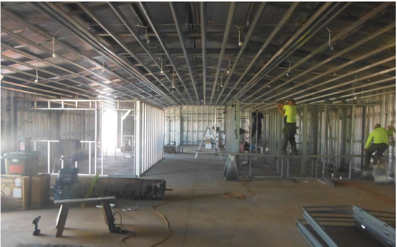
ASCC female industries shed
