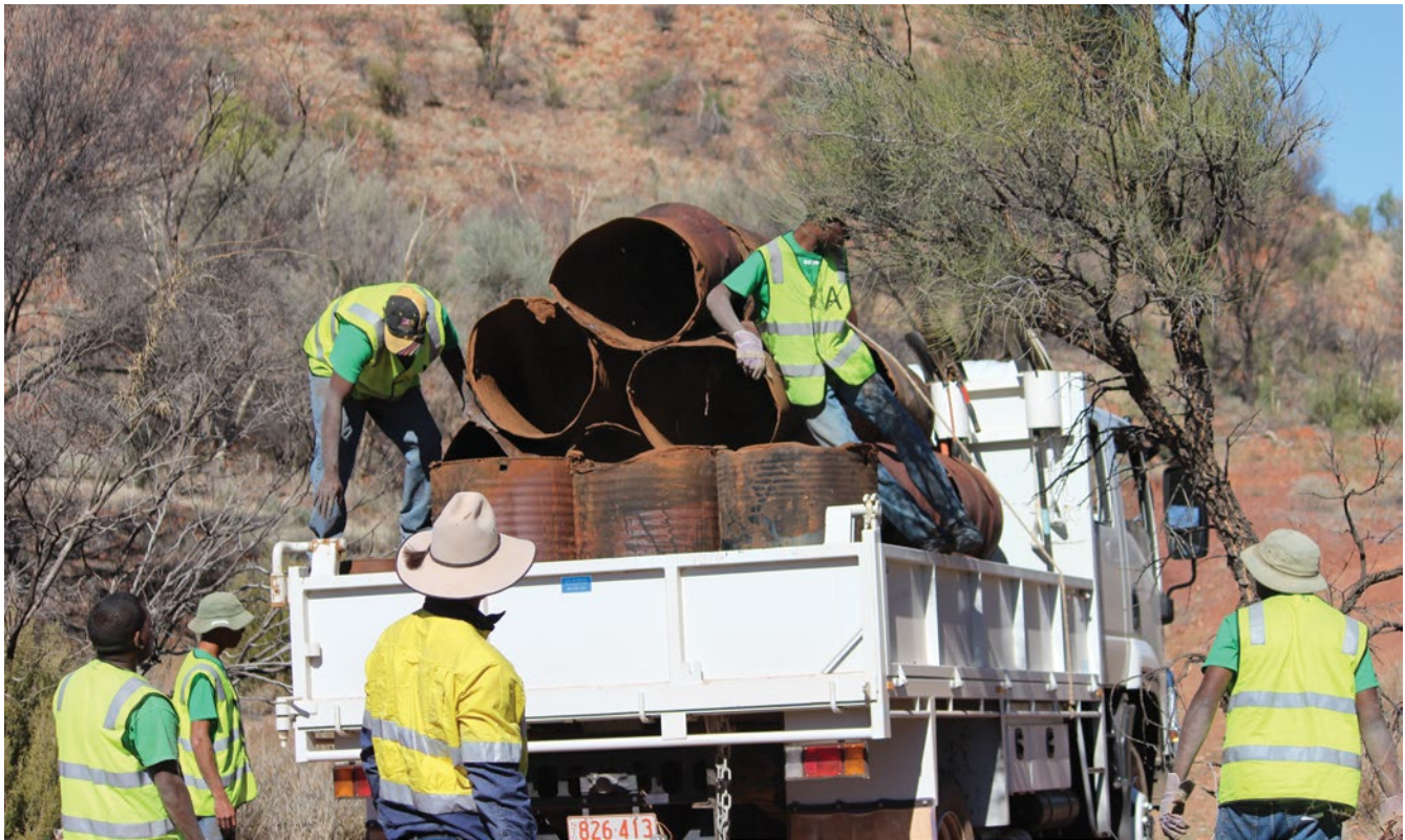
Barkly Work Camp – waste disposal
