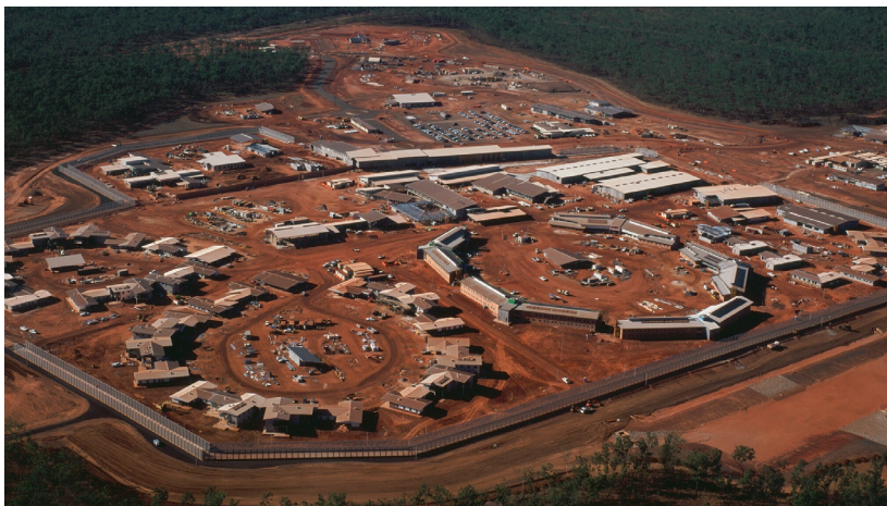
Aerial view of the Darwin Correctional Precinct.
