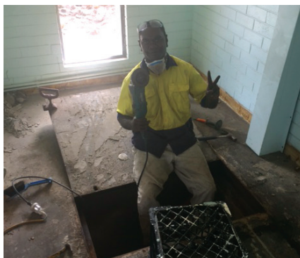
During and on completion of upgrade
