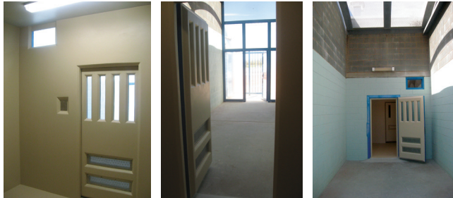
Safe Cell at Alice Springs Correctional Centre
