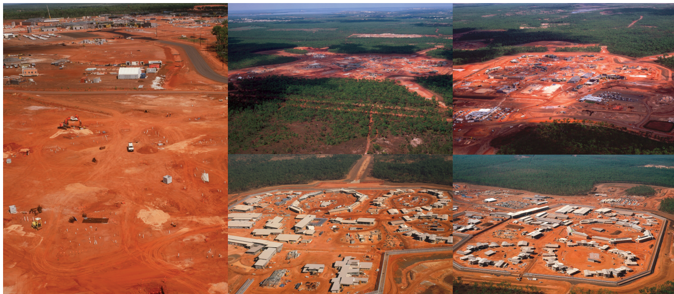
Photos: Construction of Darwin Correctional Precinct from November 2011 to November 2014
